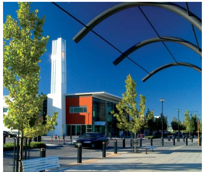
LWP head office in Ellenbrook
